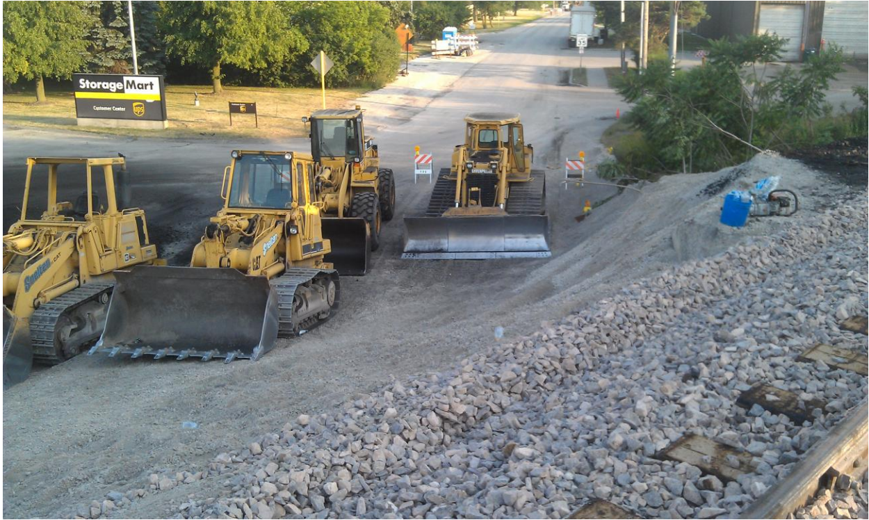
South slope looking south along Shermer Road
