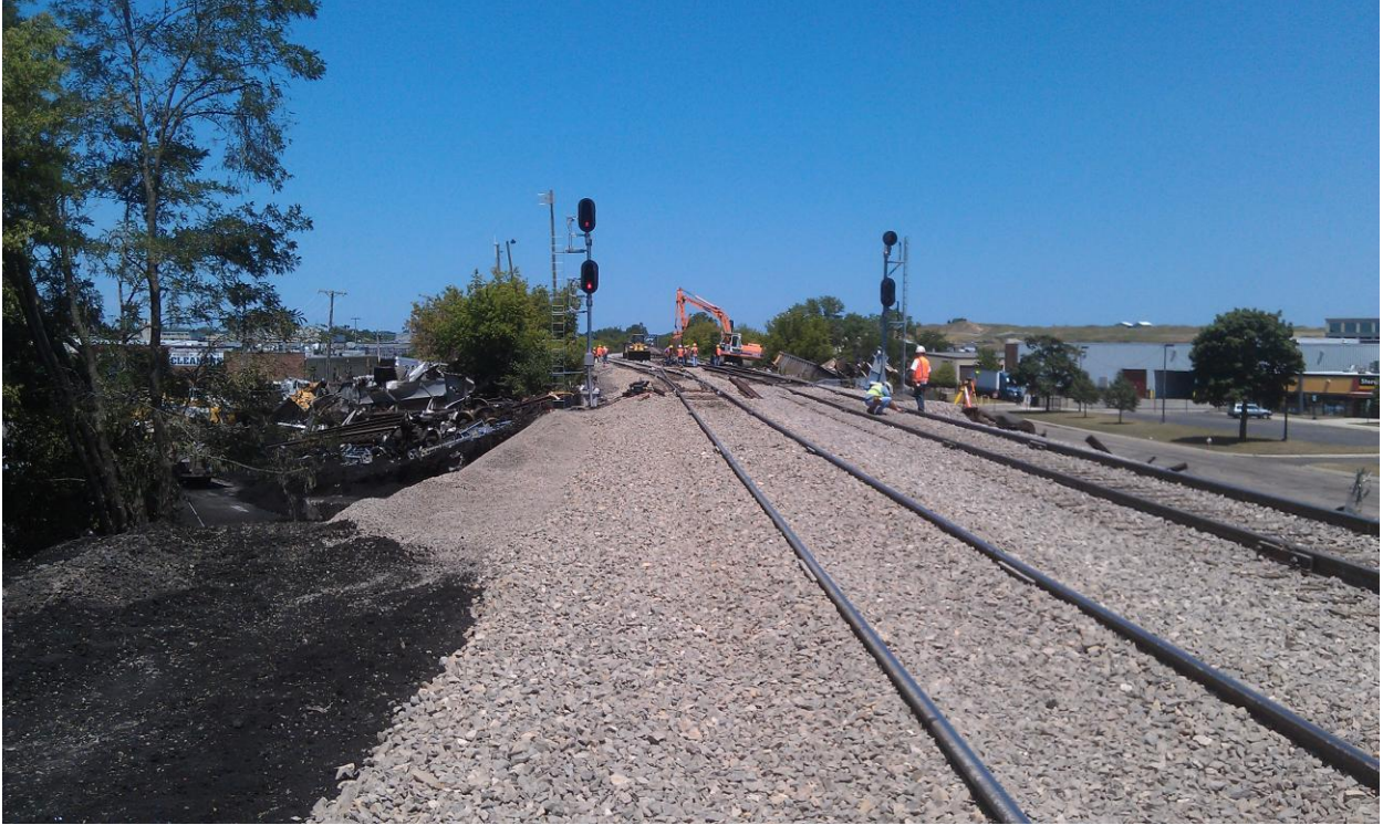
North slope looking north along Track 1
