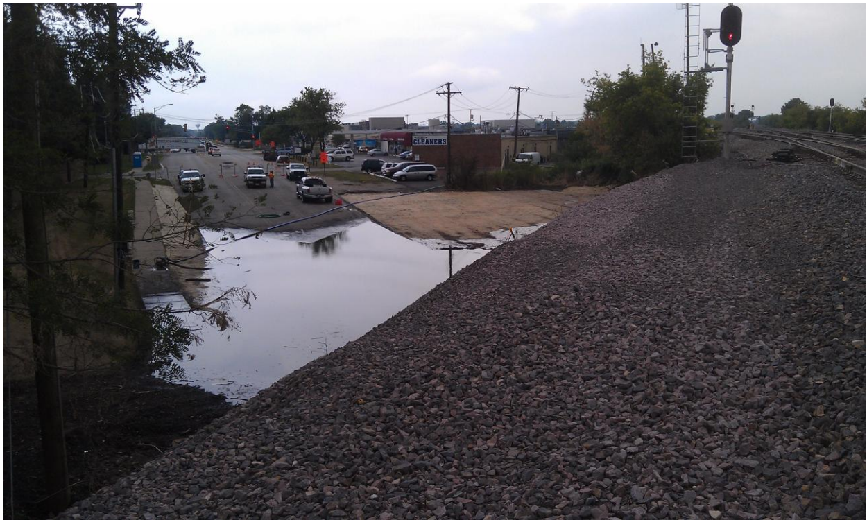
North side of Shermer Road after two inches of rain
