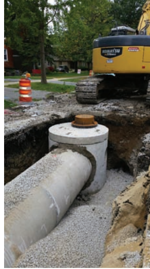
Left, a segment of 48-inch replacement pipes installed under Dewes Street. Above, inside the new pump station at Cunliff Park.
