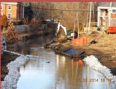
Above: Under construction, December 2014
