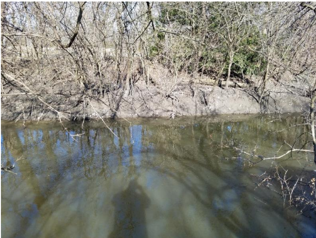
View from east bank at curve south of E. Lake Ave., looking northwest toward opposite bank
