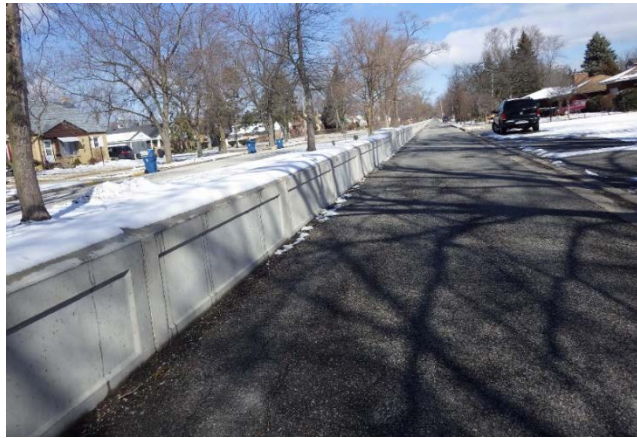
Figure 7. Concrete Block Floodwall Structure
