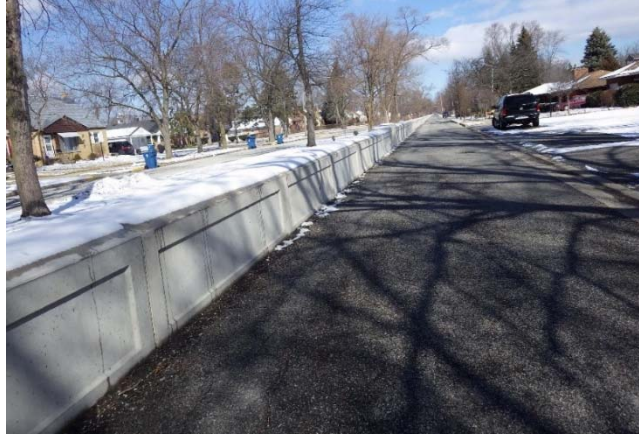
Figure 5: Concrete Block Floodwall Structure
