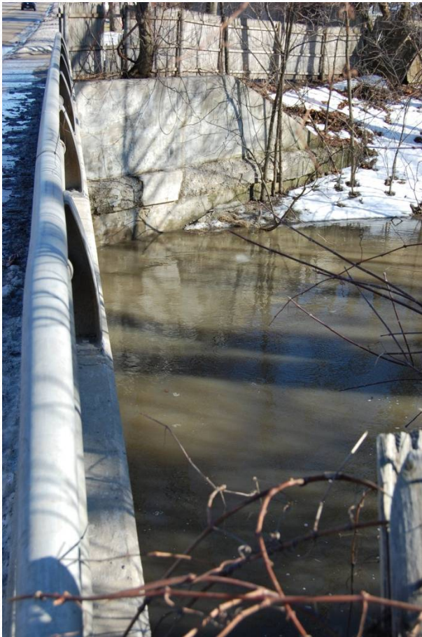
Normal State – Feb 7, 2009 Chestnut Overpass
