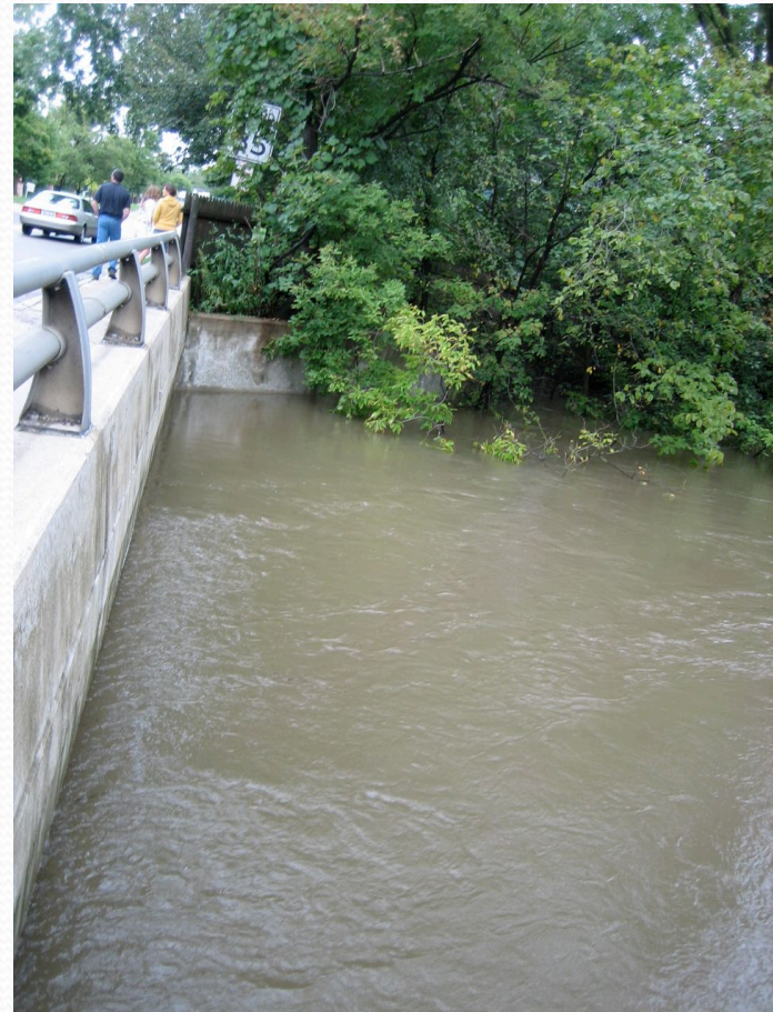
September 12, 2008 Chestnut Overpass
