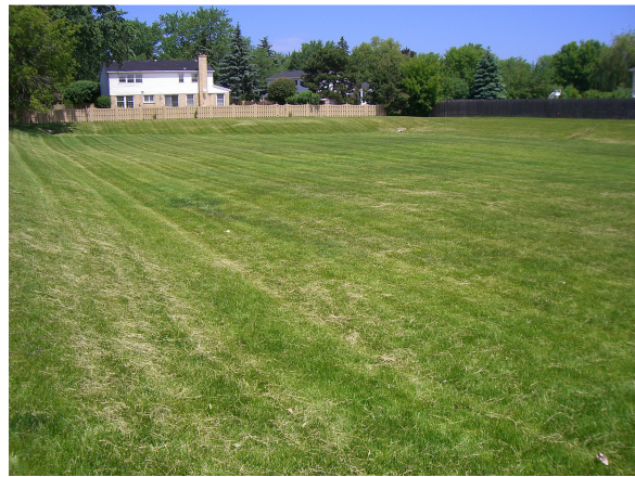
Dry-bottom detention basin (site D-3).
