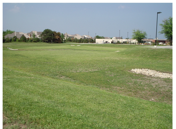
Dry-bottom detention basin (site P-1).
