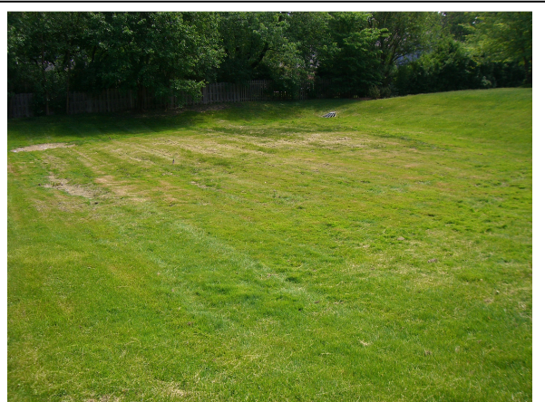
Dry-bottom detention basin (site D-2).
