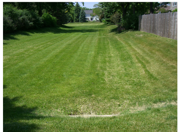
Dry-bottom detention basin (site C-5).
