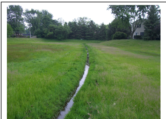
Dry-bottom detention basin (site O-4).
