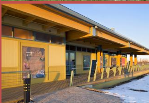
Top: Construction of the “green roof” Bottom: Interpretive displays at the Center
