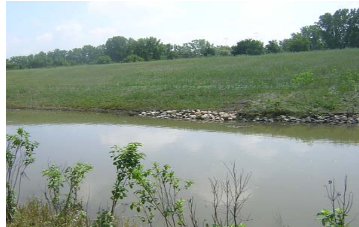
Photo 14. Bank stabilization at Lot 16
