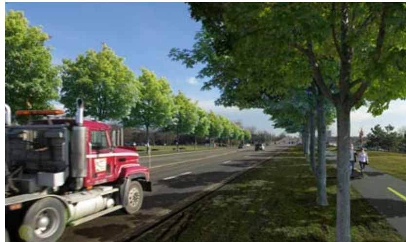
Tree planting at edge of right-of-way ensures that future road widening will leave the trees intact.
