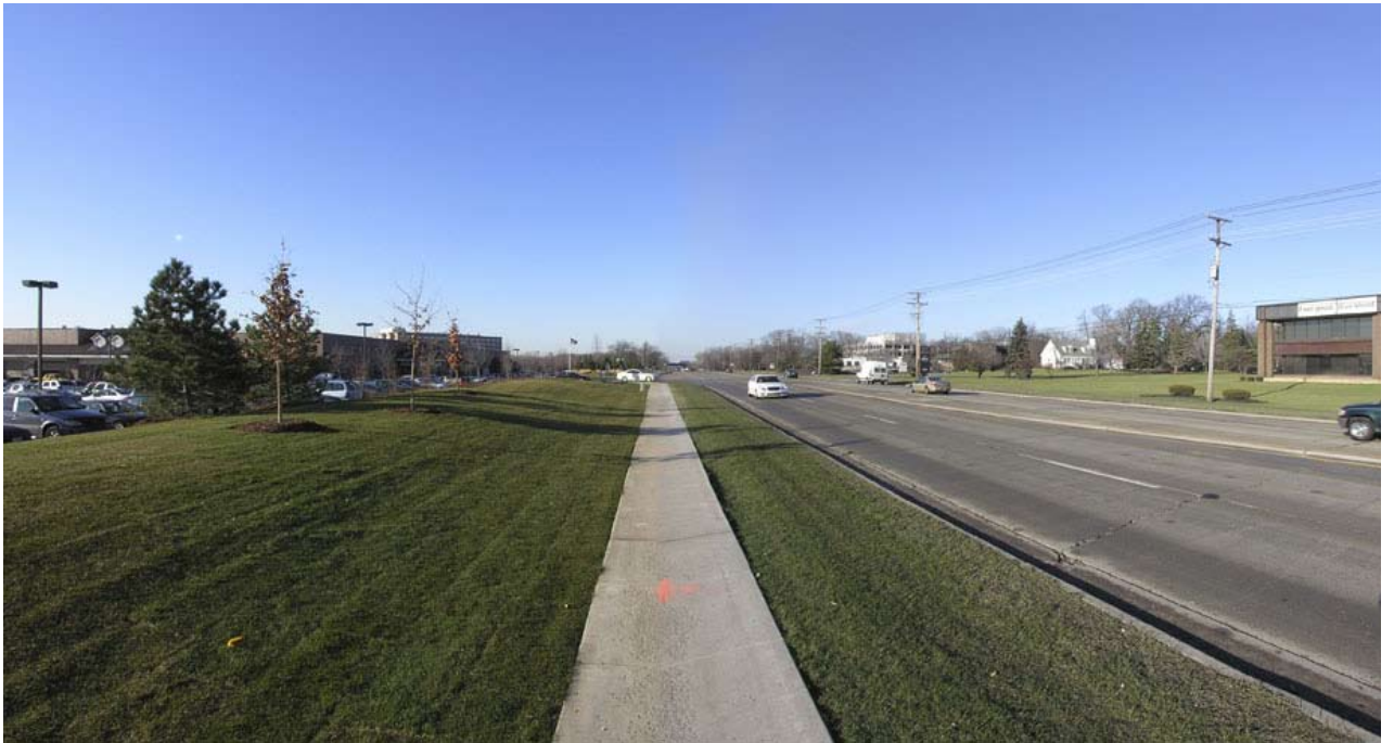
Looking north along Milwaukee adjacent to Abt Electronics.
