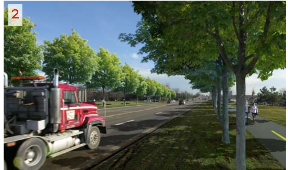
2 Improved Street Edge. Using the ultimate right-of-way line (120 feet wide), trees and a multi-purpose path are provided to enhance the edge of the street. A wide shoulder remains as the location for a future travel lane.
